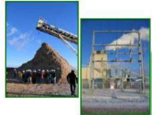
Dapp Power Plant Dapp, Alberta
