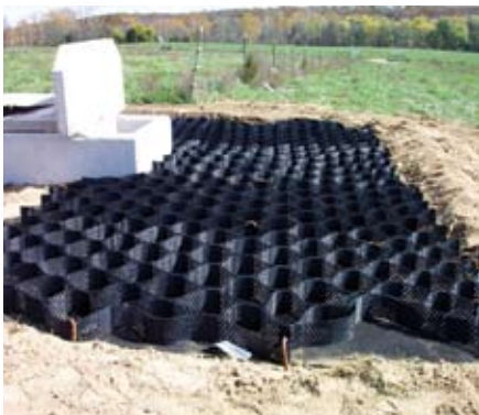
Geoweb on top of geotextile reinforces gravel pads.
