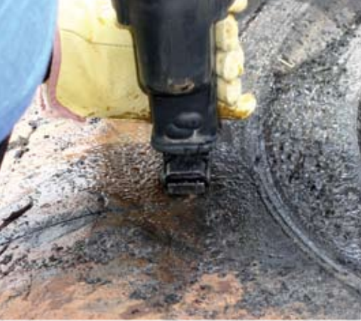
Cut the side wall from the tires.
